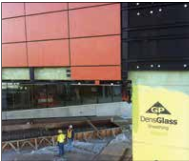
Open joints contribute to the system's self-ventilating features.
